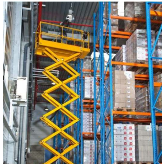
Difficult to maintain and test
