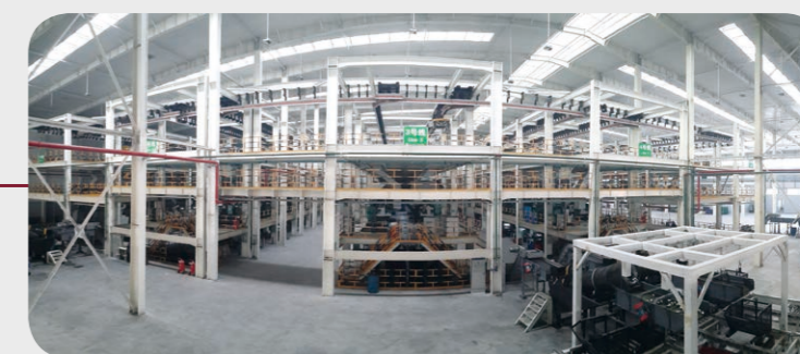
Threading, Air Pressure Test, and Anti-rust Treatment
